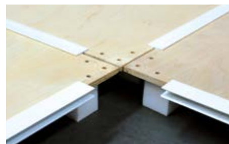
Floor and dynamic foam mounts.
