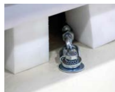
Detail of the anti-rotation kit.
